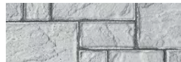
Pavers with Polymeric Haze
